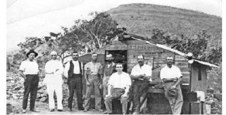
Charles in front of a worker's hut at the construction of the Wyndham Meat Works c. 1917. He is second from the right hand side of the photo.
